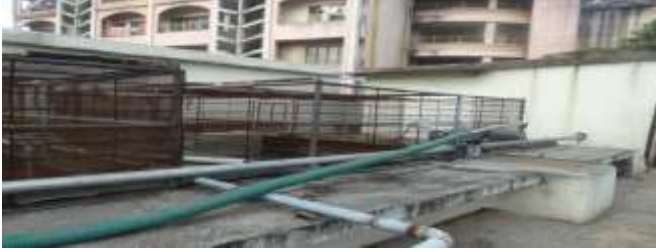
Sewage Treatment plant- I
